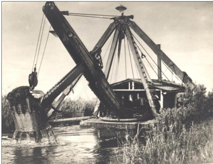
**Photo 2.** Cleaning of Dubna riverbed in 1929 with the walking water excavator “Marion” (История мелиорации ..., 2019).
